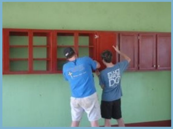
Hanging new kitchen cabinets
